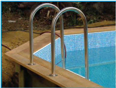
Stage 6 Top rail and internal ladder fitted
