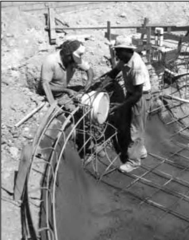
Fig. 8 BADUJET Ready for Guniting
